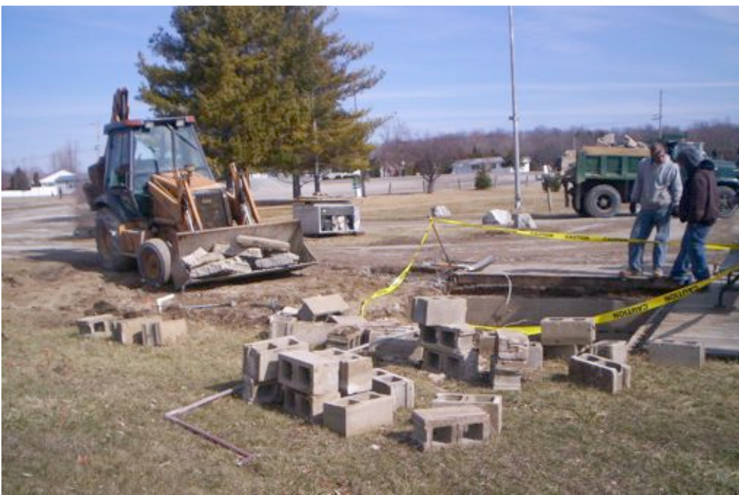
WORK ON THE MARINA CONTINUES
